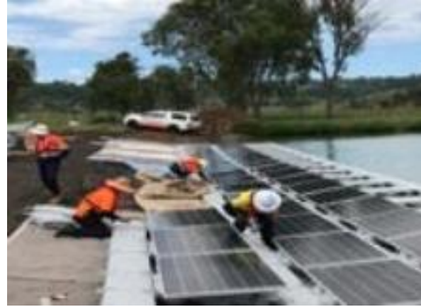
Floating Platform Assembly
